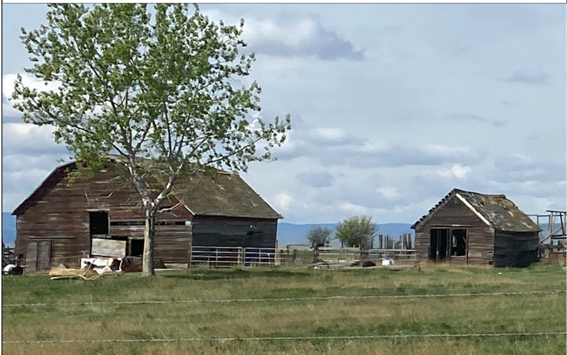
Photo 4: Additional view of the on-site farmstead, noting wooden structures in disrepair.
