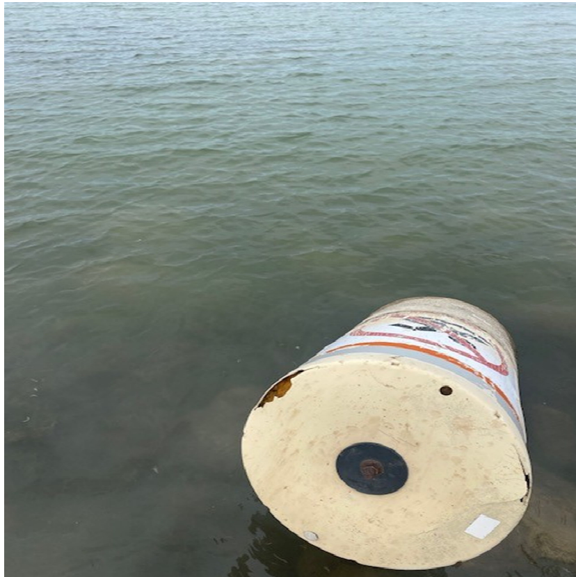
Pine Coulee Raw Water Intake Marker
