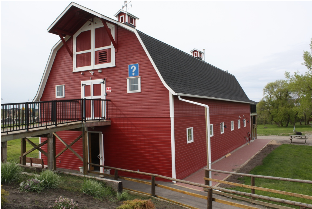
Shepherd's Park Barn Community Space Exterior, High River, AB
