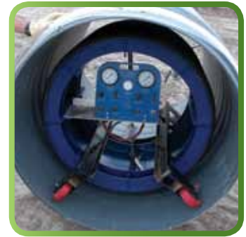
Joint Isolation Test
