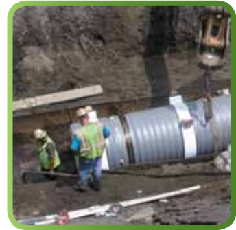
Sliplining and Trenchless Applications
